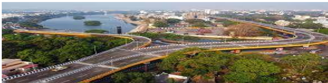
Figure – 3 Chennai to Cuddalore - State Highway\
