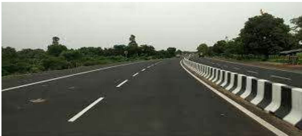
Figure 2 - The Mehsana – Himmatnagar State Highway
