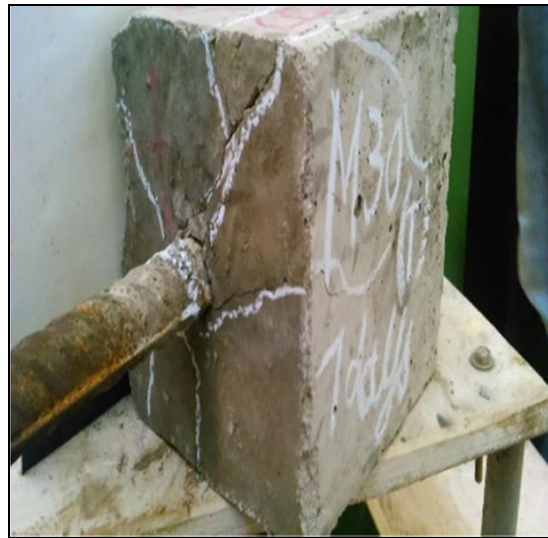
b. Cube embedded with steel rod after Testing
