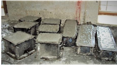
casting of samples (cubes and prisms)
