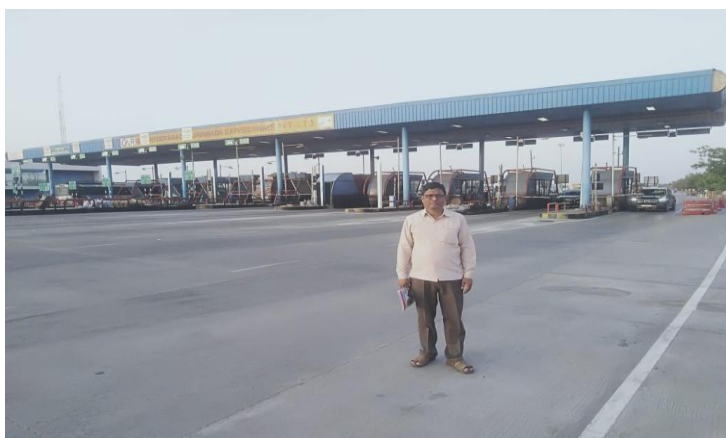
Fig 4 View of Korlapahad Toll Plaza on NH65
