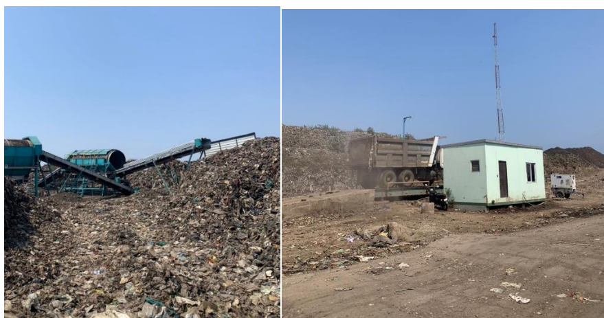
Fig. 1(a), 1(b) ongoing biomining process at site
