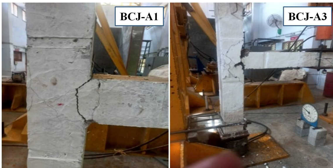
Figure 7(a) Crack patterns of control specimens
