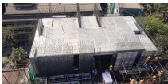
Figure 04 Slab decking
