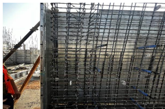
Figure 02 Erection of wall panel
