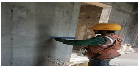
Figure 06 Removing wall tie
