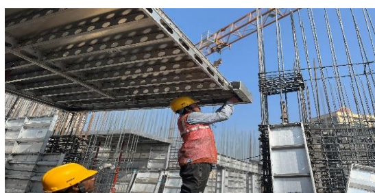
Figure 05 Fixing of deck panel
