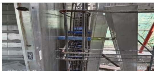
Figure 03 Erection of wall tie
