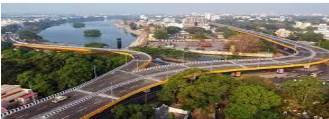
Figure – 3 Chennai to Cuddalore - State Highway
