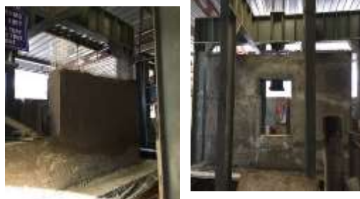
Fig.3 Finished wall panel
