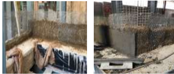
Fig.2 (c) Earth and straw filling, compacting and plastering of wall panel
